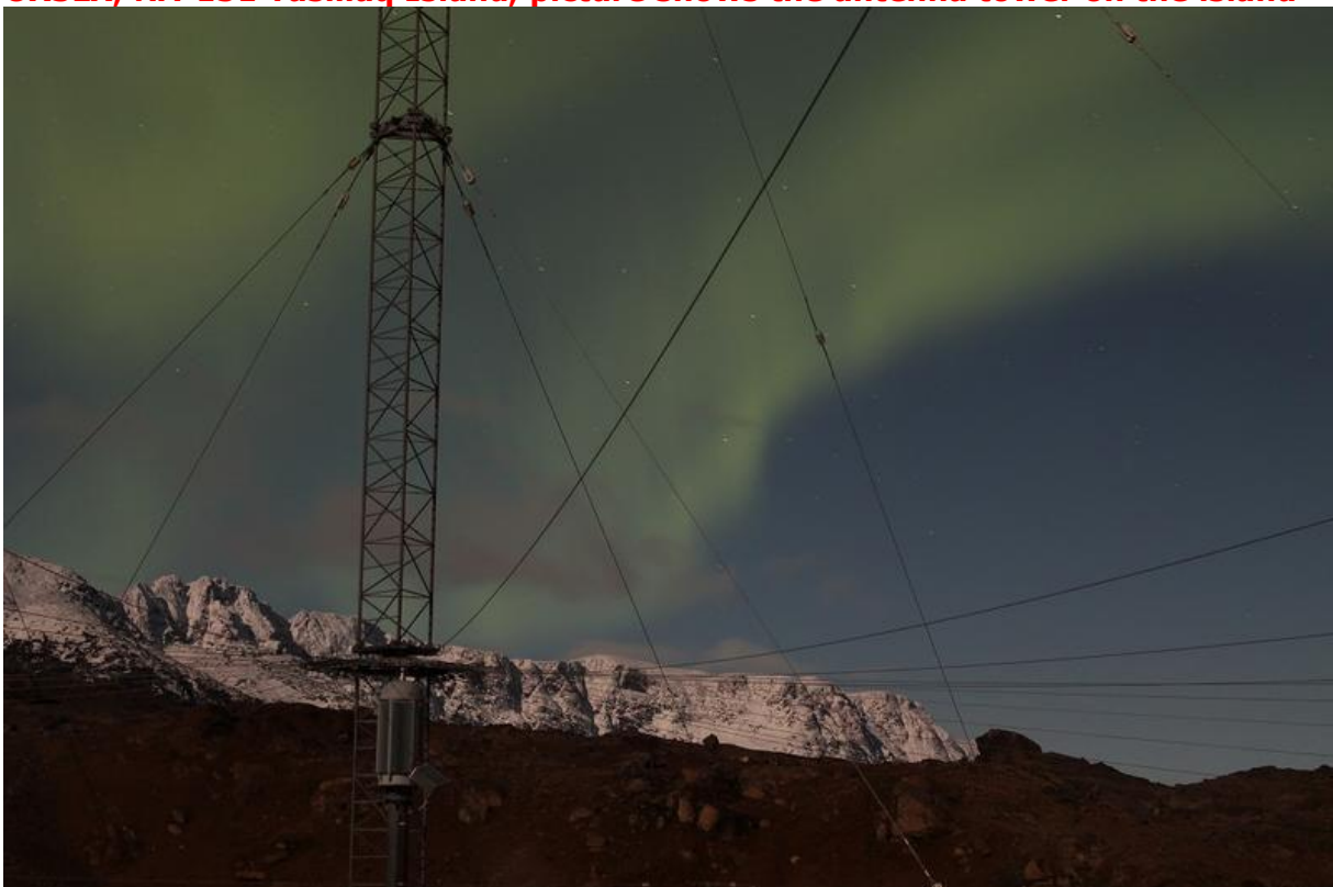
OX3LX, NA-151 Tasiilaq Island, picture shows the antenna tower on the island
